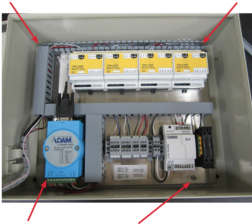
Back plane assembly securing bolt locations
